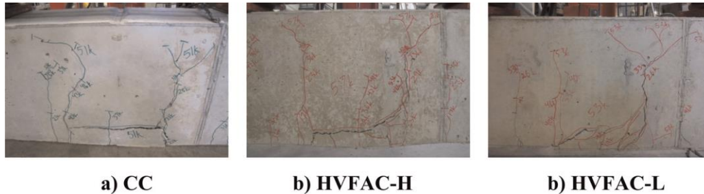
FIG. 3 – Crack pattern of the beams at bond failure.
