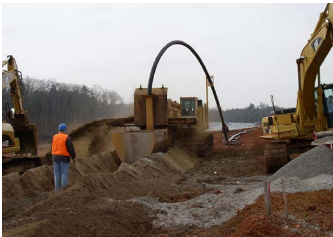
Figure 6: Slurry Wall Installation
