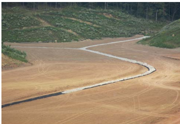
Figure 11. Conveying channel riprap revetment installation.
