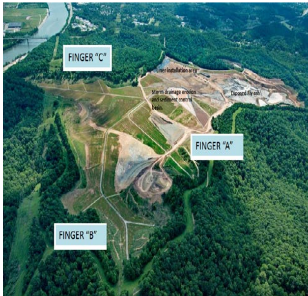
Figure 14. Completed cap system over fingers including erosion and sediment basin for non-contact storm water management, liner installation of middle section, exposed fly ash towards pumping system handling contact storm water.
