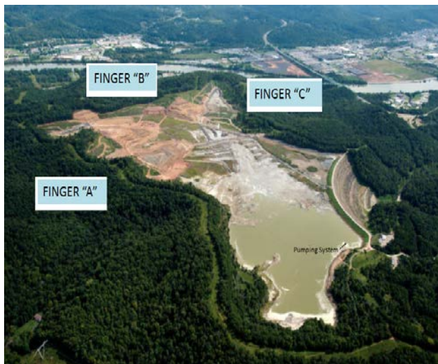
Figure 5. Free water drainage and removal.
