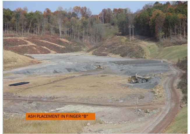
Figure 8. Placements of excavated fly ash fill to achieve desired subgrade level.
