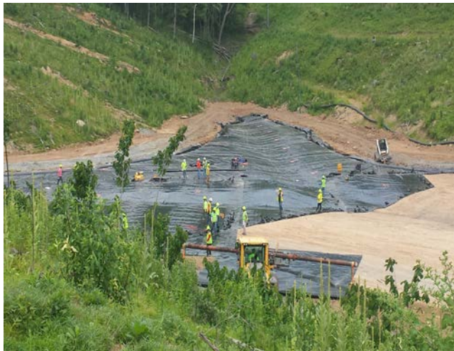
Figure 9. Liner installation
