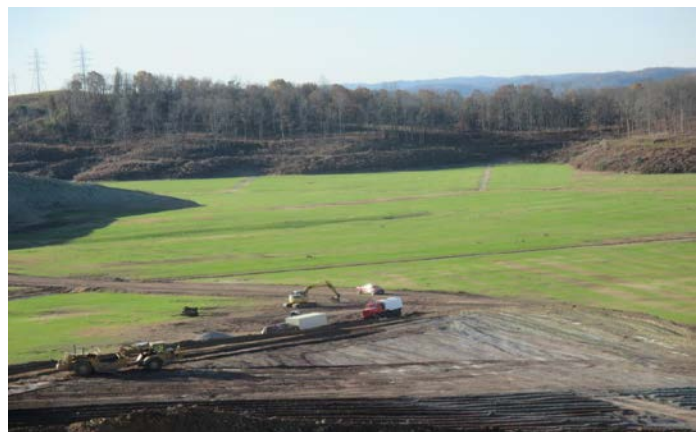
Figure 12. Vegetative cover of cap system.
