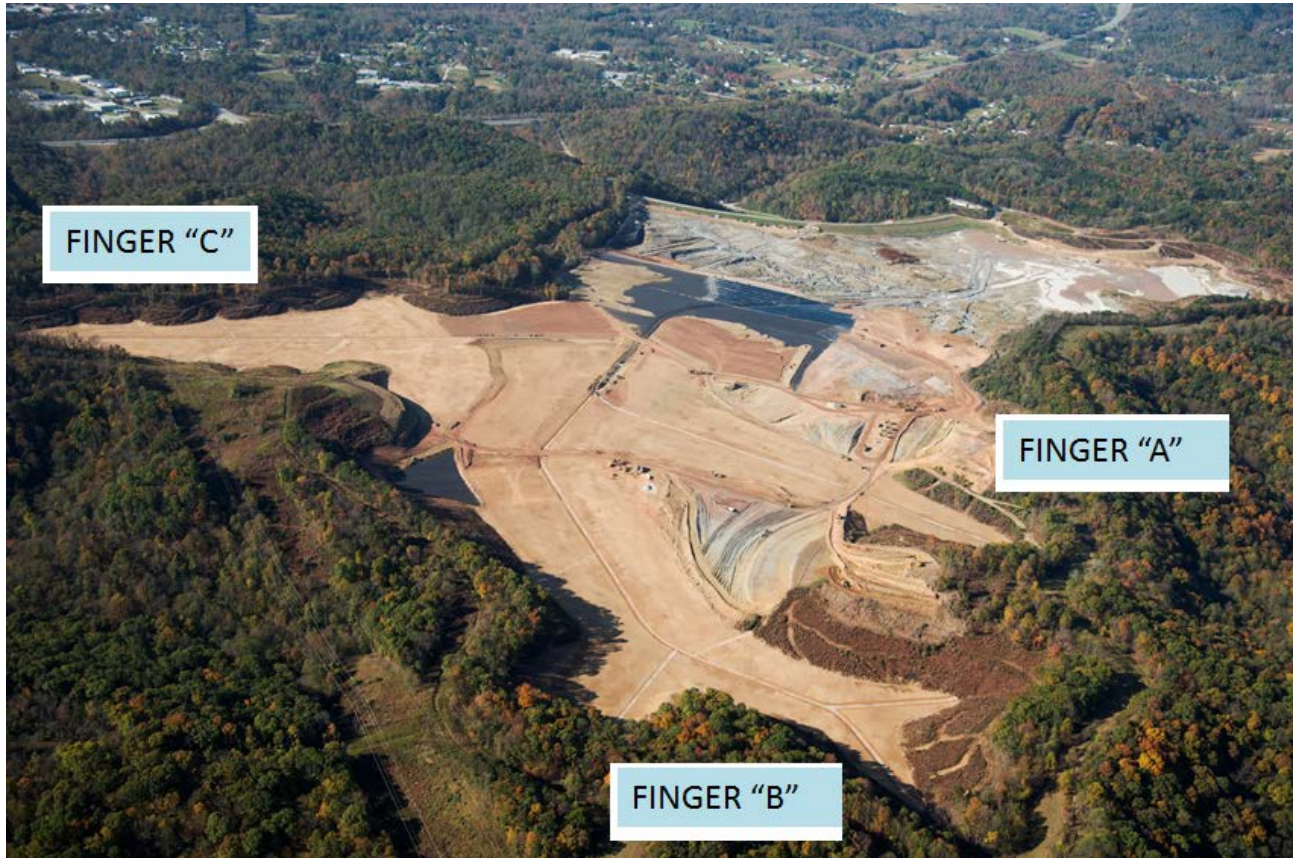
Figure 13. Progress of installation of cap system
