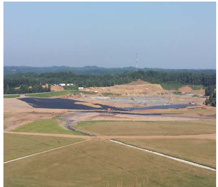
Figure 14. Completed cap system over fingers including erosion and sediment basin for non-contact storm water management, liner installation of middle section, exposed fly ash towards pumping system handling contact storm water.
