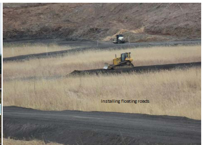
Figure 4. Installation of floating roads over exposed fly ash subgrade.
