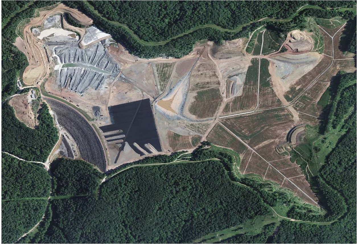
Figure 16. Work completed as of June 2016.
