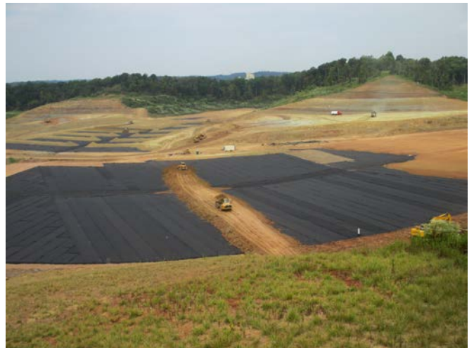
Figure 10. Installation of liner's protective cover including cushion fabric.
