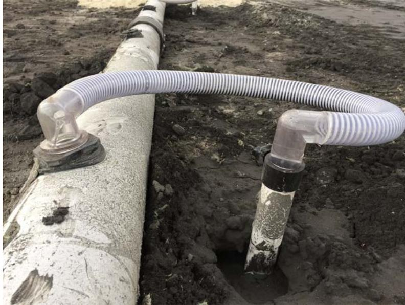
**Pictured: Significant flow and low turbidity water can be produced from properly constructed wellpoints in ash.**
