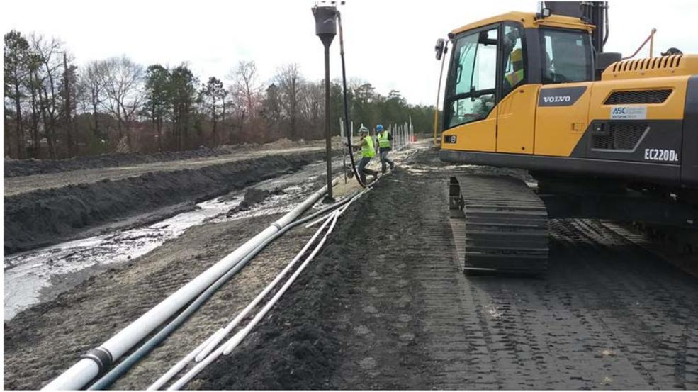
**Pictured: wellpoints installed along an existing rim ditch to stabilize ash for fine grading and liner**
