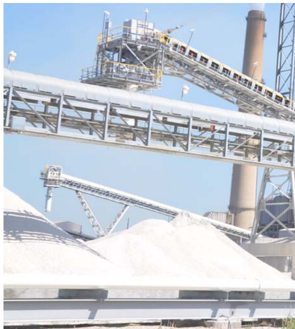
Photo 2. Radial stacker discharge to pad.
