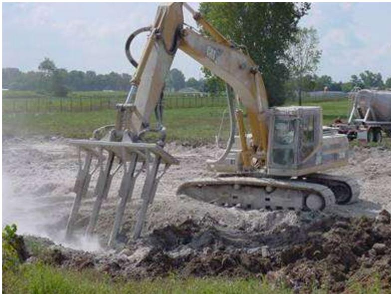
Excavator Injecting Lime Into Pond and Mixing
