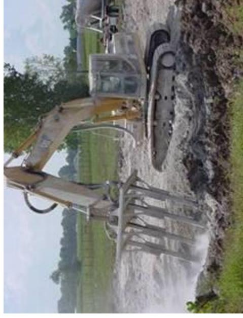
Deep mixing injector – follows stabilization across pond
