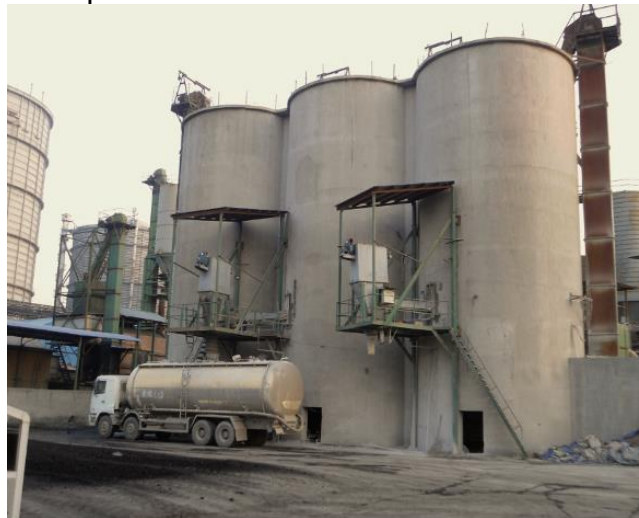
Figure 10 Use DFGD as Mixture in JINSHICHUAN GGBS Plant, Nanjing
