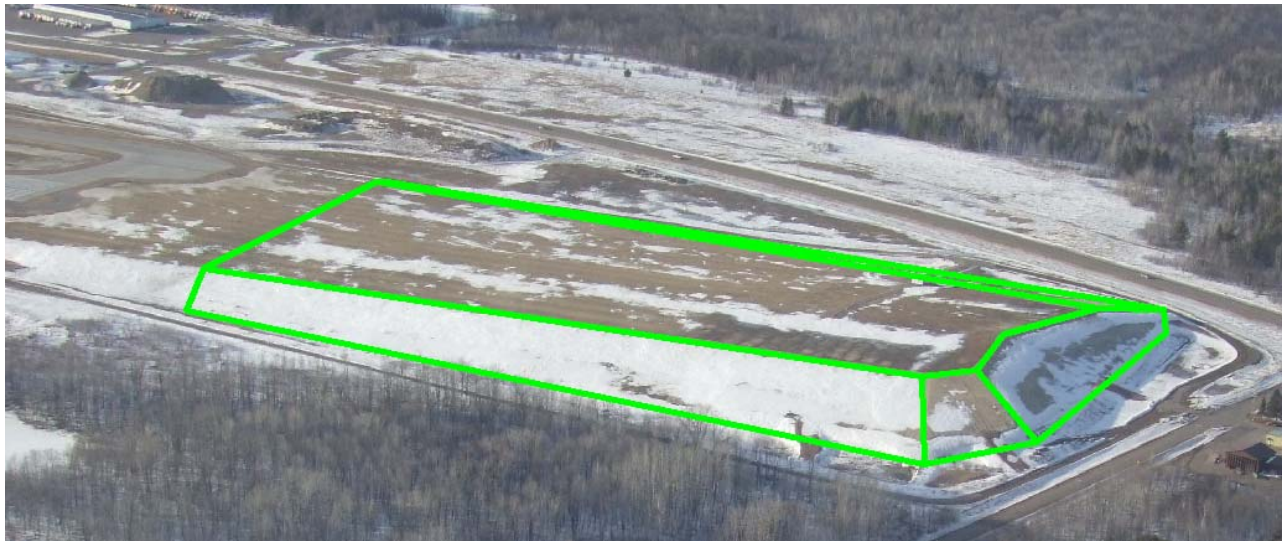
Photograph 1 – CWA Beneficial Reuse Project on February 19, 2011
