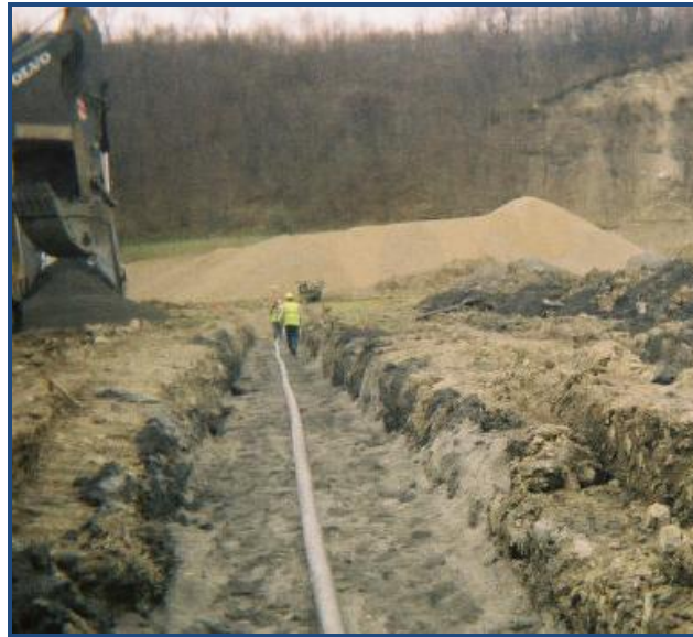
Figure 2a: Settlement “Profiler” System Installation
