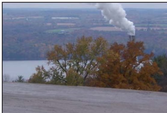
Covered Flyash Landfill
