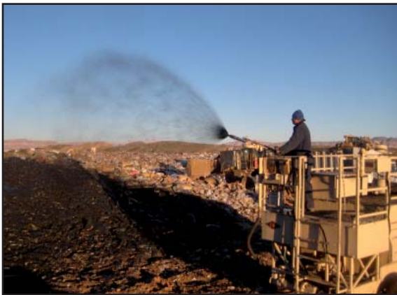
MSW Landfill Test Application
