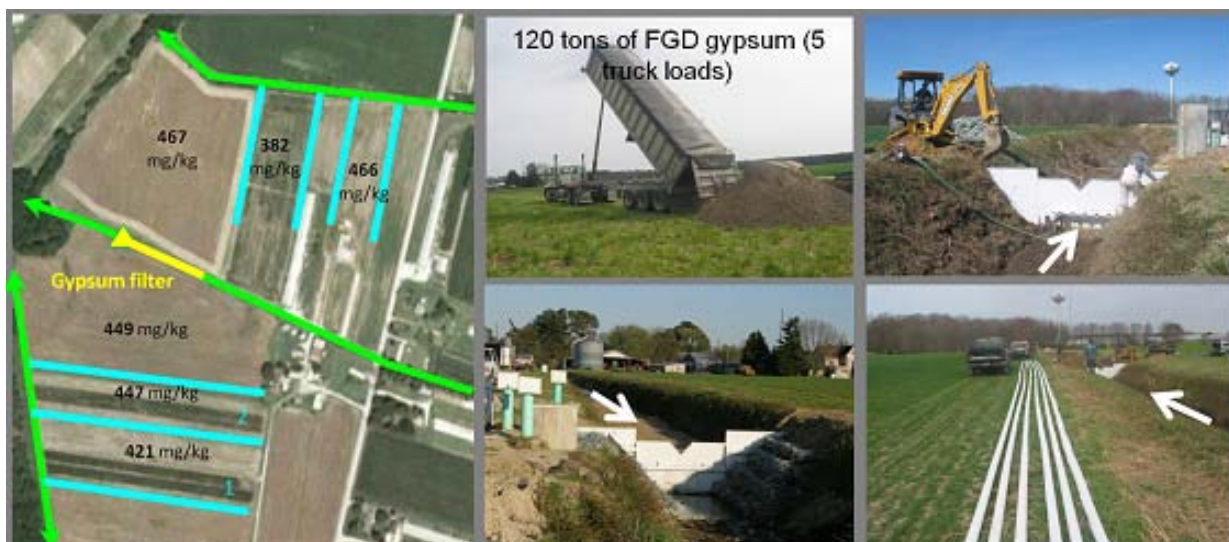
Figure 2. Clockwise from left: Location of the gypsum filter; 120 tons of FGD gypsum was used in construction; a weir impedes ditch flow and measures overflow (white arrows show direction of flow); six 10 cm tile lines (30 m long) attach to the manifold in front of the weir; tile lines embedded in sand are sandwiched in FGD gypsum above and below; filtered effluent is routed underground around the weir and through flow and concentration monitoring instruments before release downstream.
