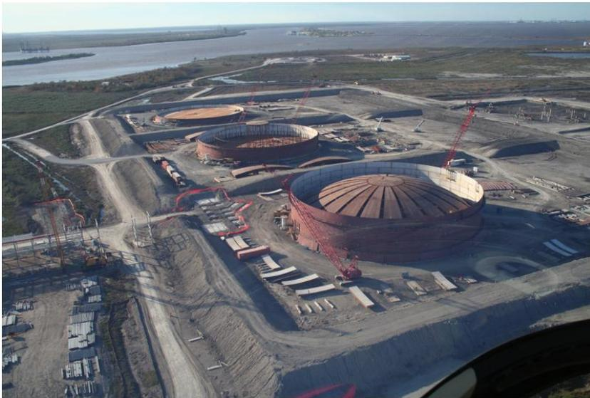
Figure 2: Hurricane protection levees were constructed from stabilized dredge spoils and we placed on a 2:1 slope. No failures, significant erosion, or structural problems have been identified in the 3 years since construction.
