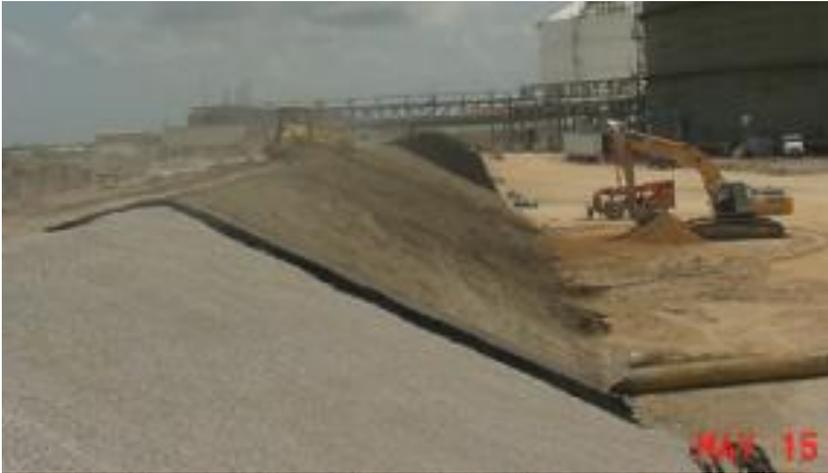
Figure 1: Dredge spoils with a strength of zero were stabilized to support a 2:1 slope, retain an ultimate strength in excess of 25 psi when measured using an unconfined compressive strength test.
