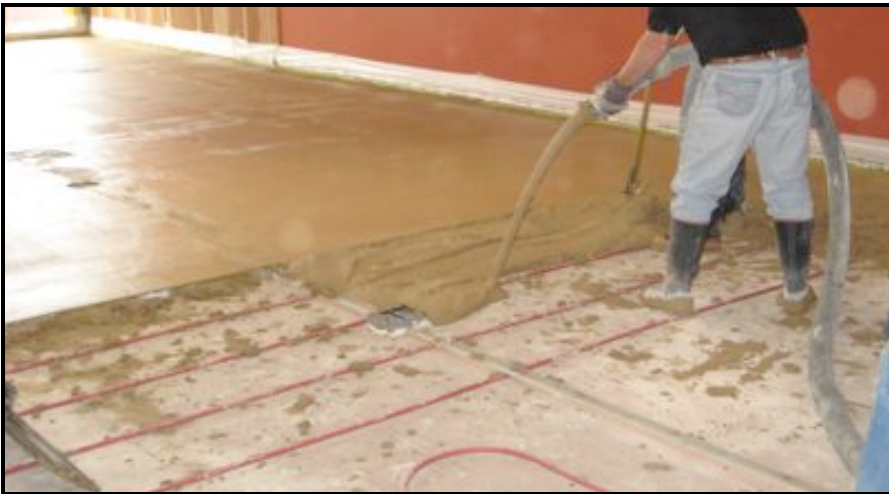
Figure 3: Placement of Glass Aggregate Mix via a Line Pump (Billings Commercial Building)
