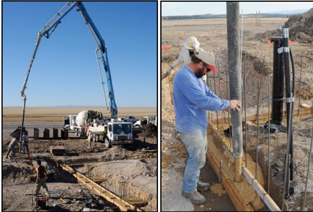
Figure 5: Pumping 100% Fly Ash Concrete with Traditional Aggregate (Lewistown, MT)
