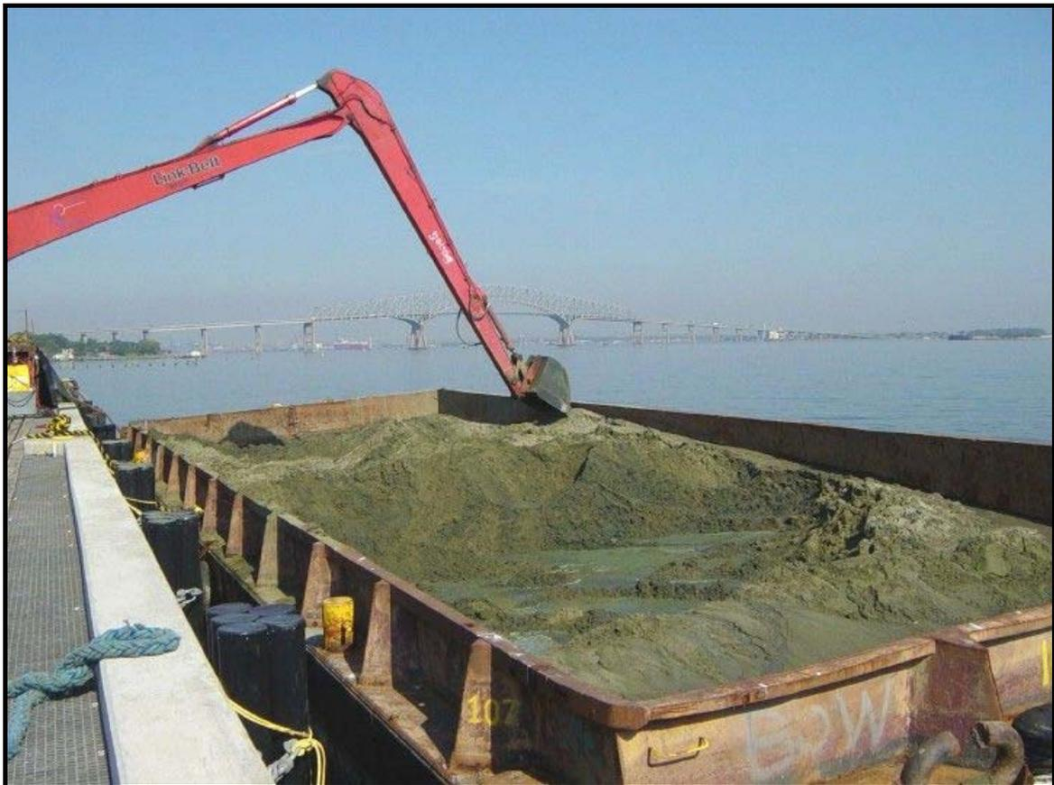
Figure 2. Cox Creek CDF Barge Unloading
