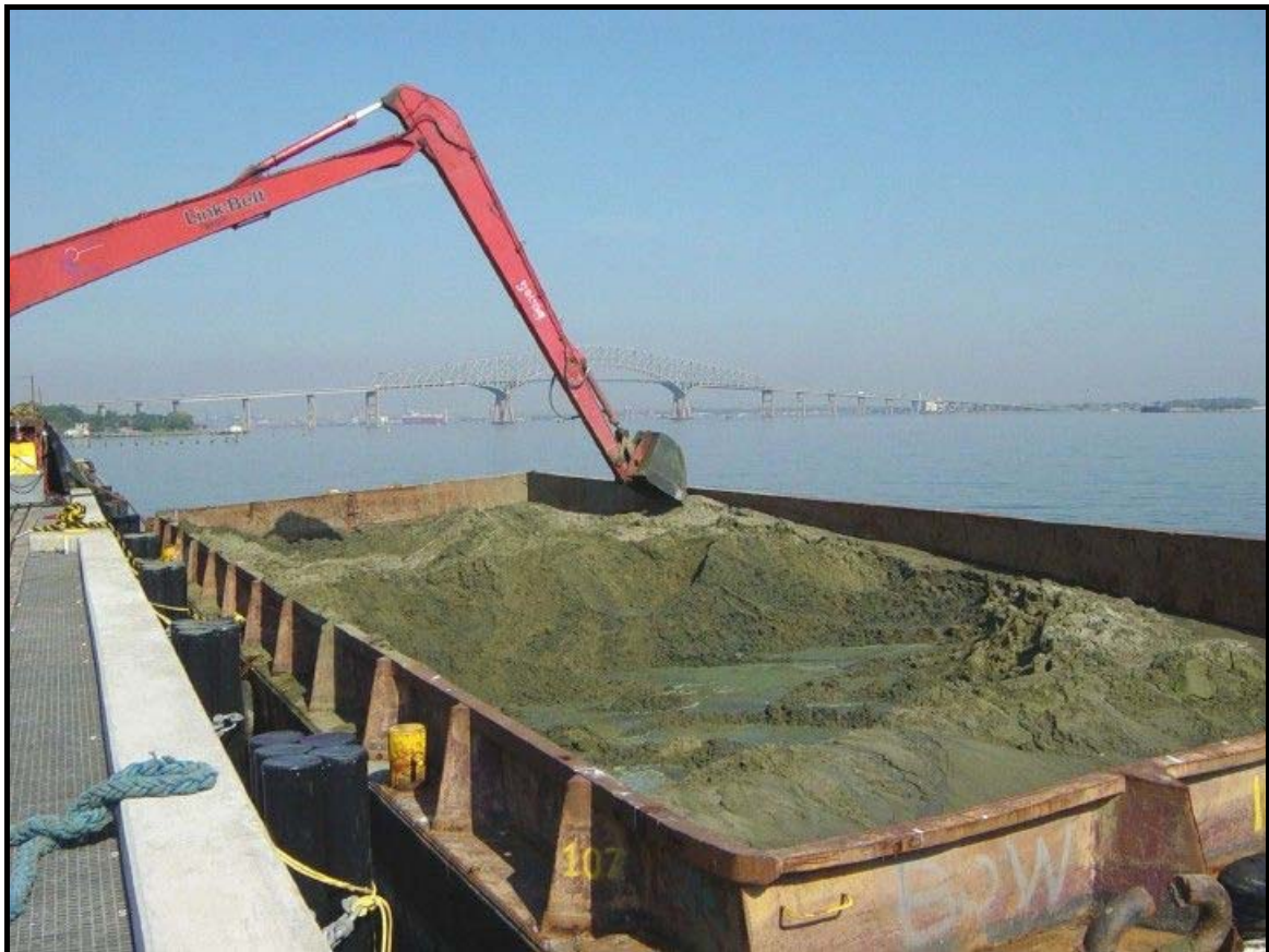
Figure 2. Cox Creek CDF Barge Unloading
