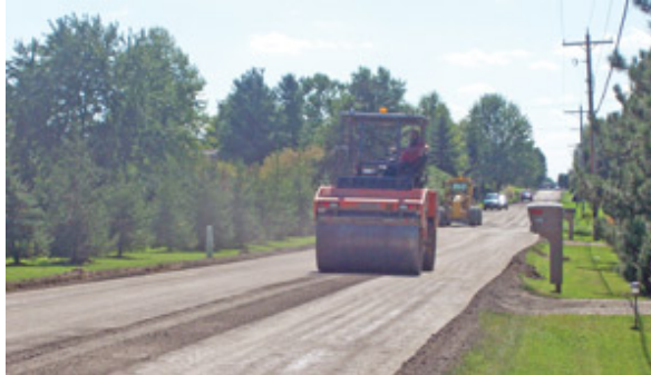
Fig. 3 Compaction of FDR base layer
