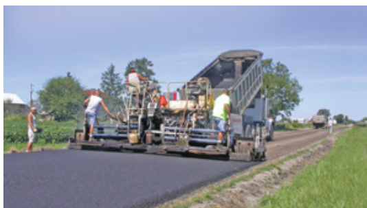
Fig.4 Resurfacing with hot mix asphalt
