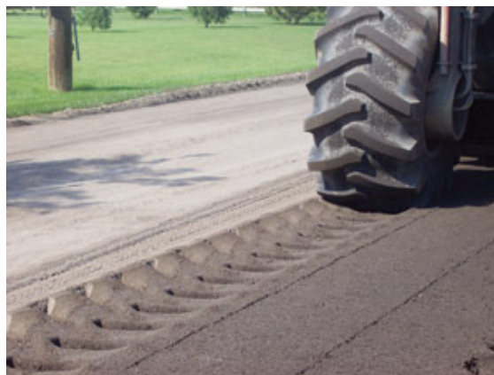
Fig. 2 Blending fly ash with pulverized base material
