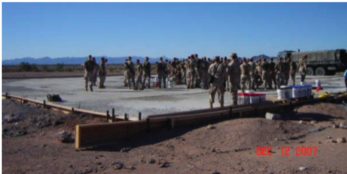
Figure 1. Marine Core Air Base Concrete Installation
