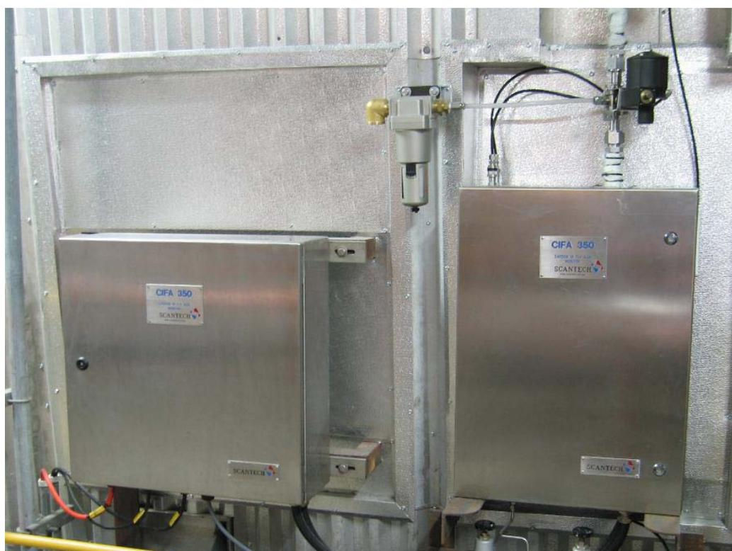
Figure 1. - CIFA350 Electronics Module and Measurement Module on a Duct
