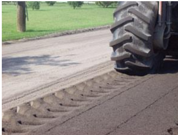
Figure 1: Blending fly ash with pulverized base material
