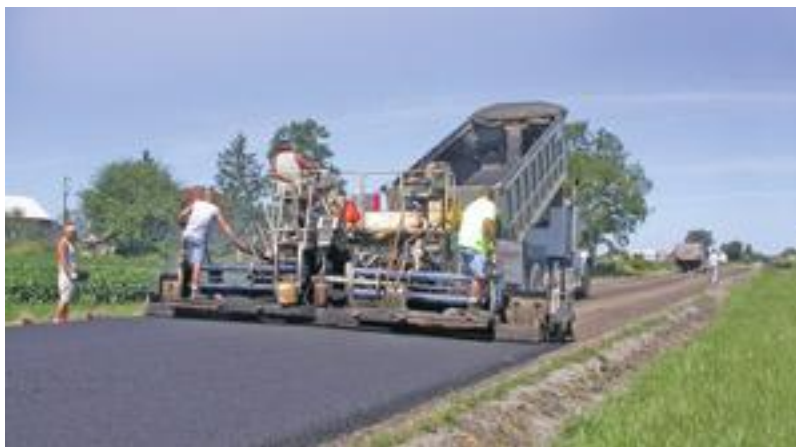
Figure 3: Resurfacing with hot mix asphalt in Warren County.
