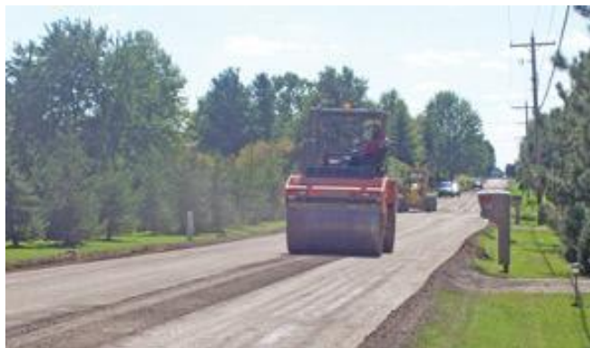
Figure 2: Compaction of the FDR base layer in Delaware County.
