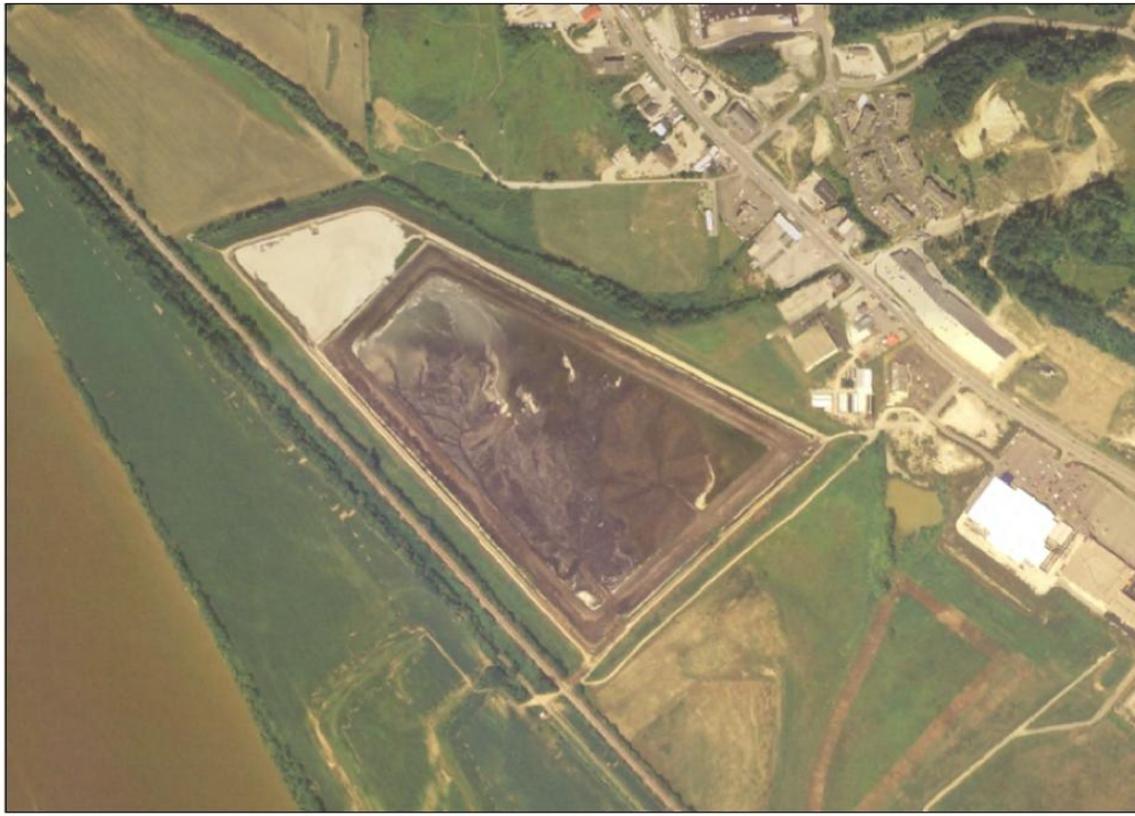
Figure 15. Fly Ash Storage pond – Elevation 518' Dam Raising
