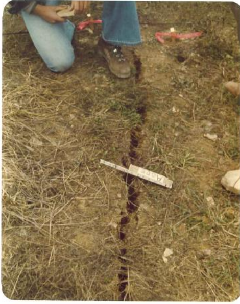
Figure 5. Tension Cracks on an area near the west abutment of the original dam
