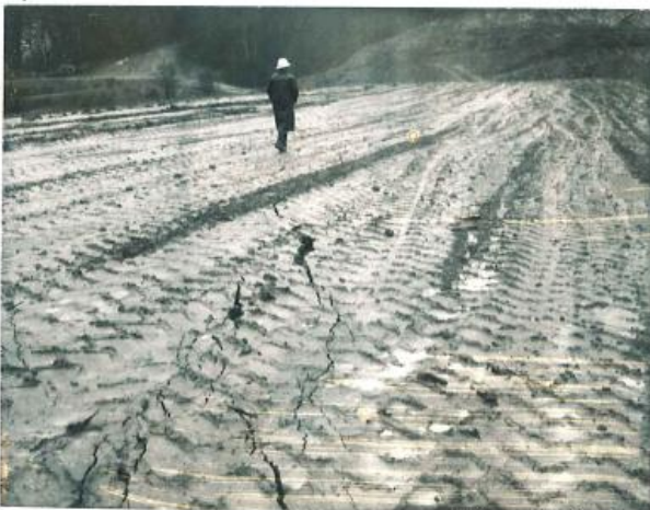
Figure 4. Tension Cracks on the Downstream Embankment of the Dam
