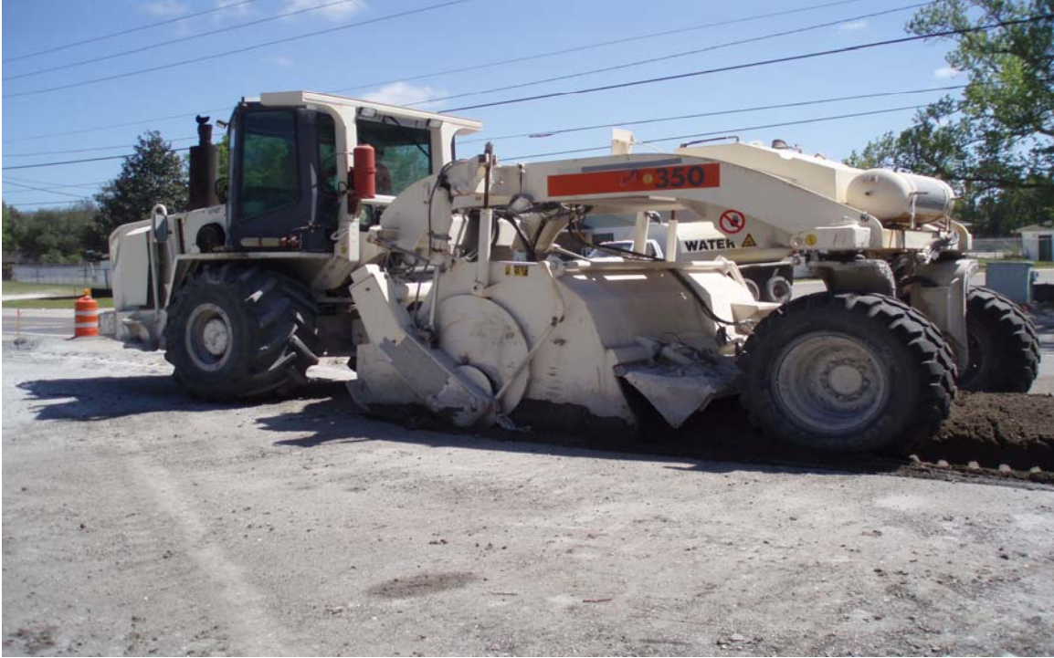
Figure 8. Mixing of EZ-Base™ Using a Typical Rotary Tiller/Mixer.
