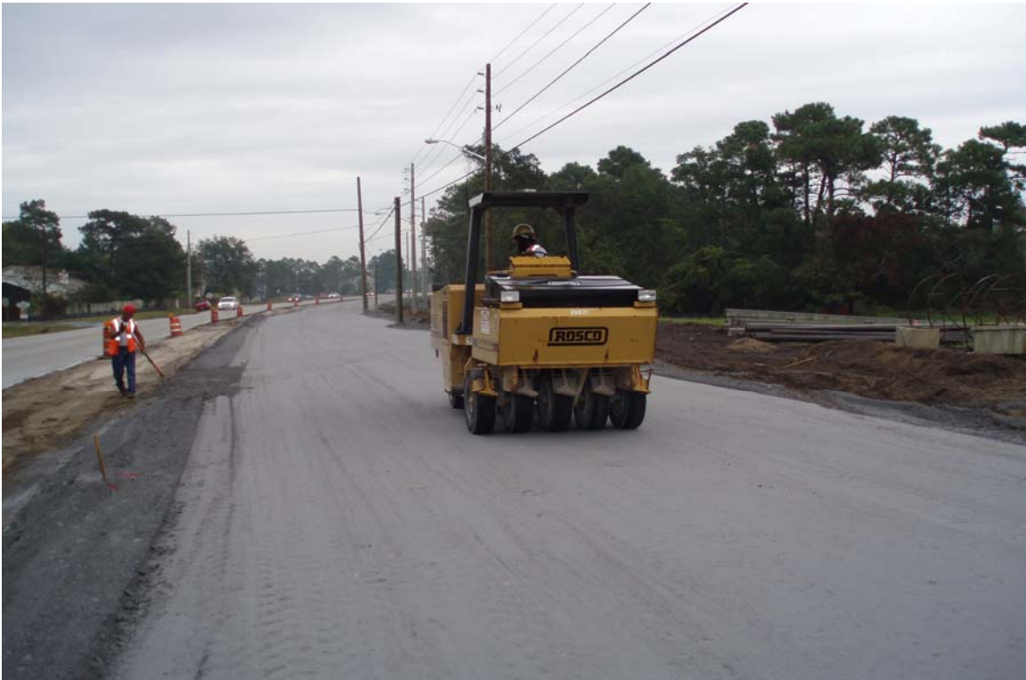
Figure 9. Compaction of EZ-Base™ Using a Pneumatic Tired Roller.
