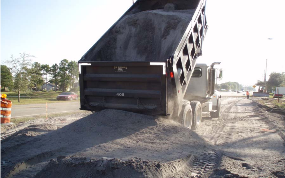
Figure 6. Delivery of EZ-Base™ to the Project Location.
