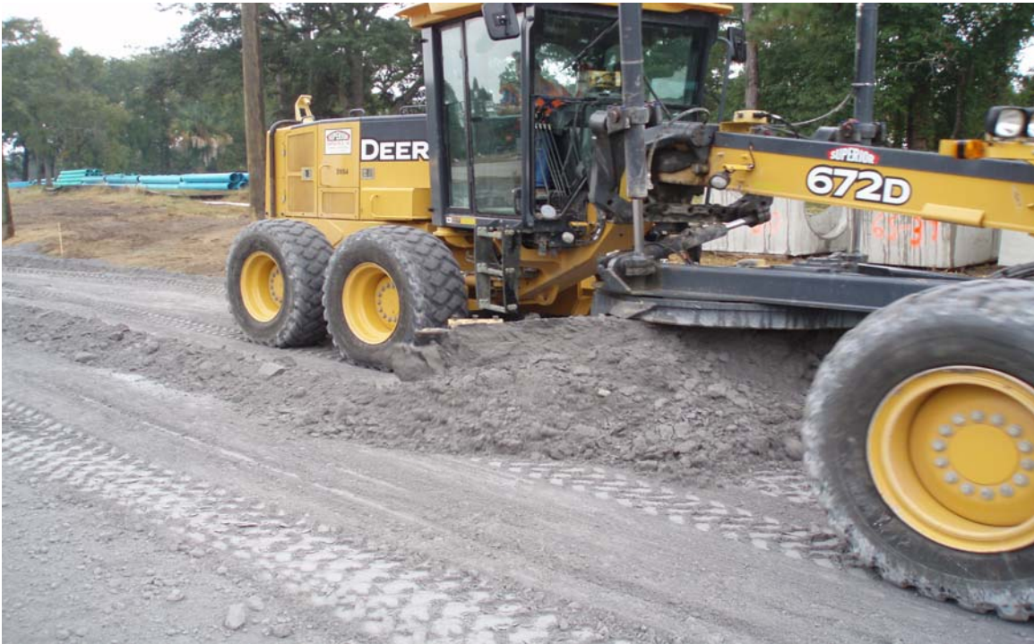
Figure 7. Spreading of EZ-Base™ to the Prescribed Mixing Thickness.
