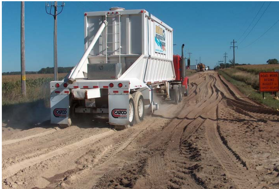
Fig. 2. Spreading of fly ash on gravel road with lay-down equipment
