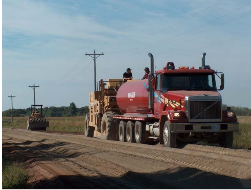
Fig. 3. Mixing process of fly ash, road-surface gravel, and water by a reclaimer (compaction is performed right after mixing by tamp-foot compactor seen in the background).
