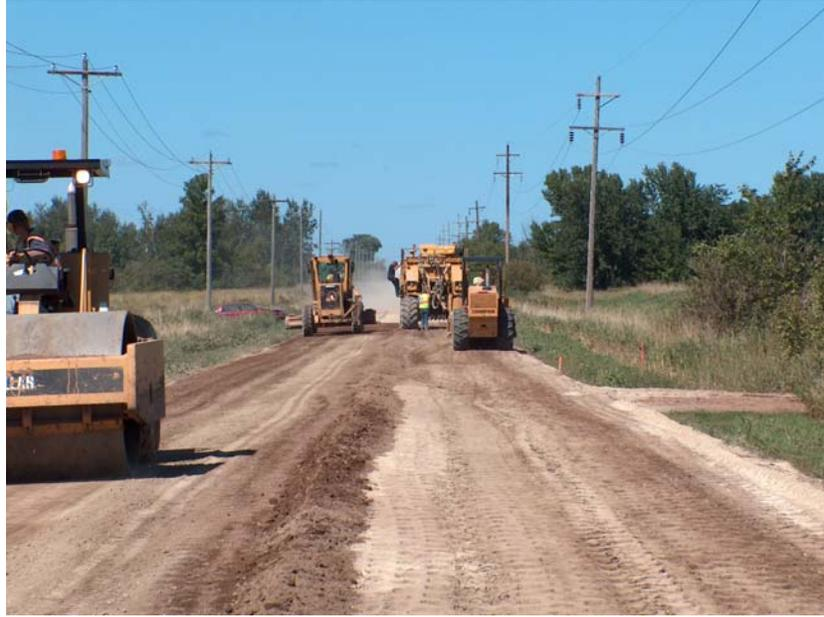
Fig. 1. Gravel surfaced County Road 53 being stabilized in situ with fly to form a firm base to for asphalt pavement
