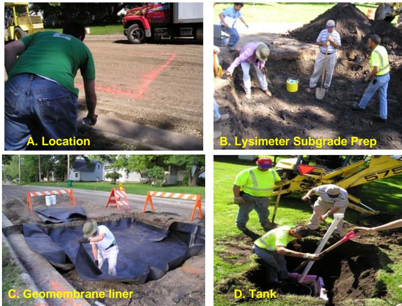
Fig. 6. Construction of pan lysimeter under 7<sup>th</sup> Avenue before fly ash stabilized base is constructed and the street is paved. Lysimeter collects percolating water through the pavement and fly ash stabilized base for quantity and quality determination.
