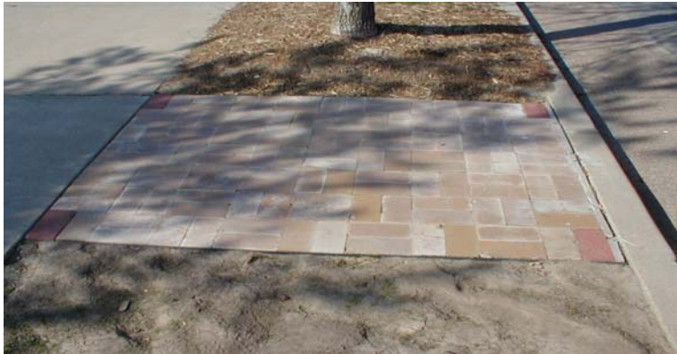
Figure 3 Compacted fly ash bricks tested for use as walkway pavement on the campus of University of Missouri-Columbia.
