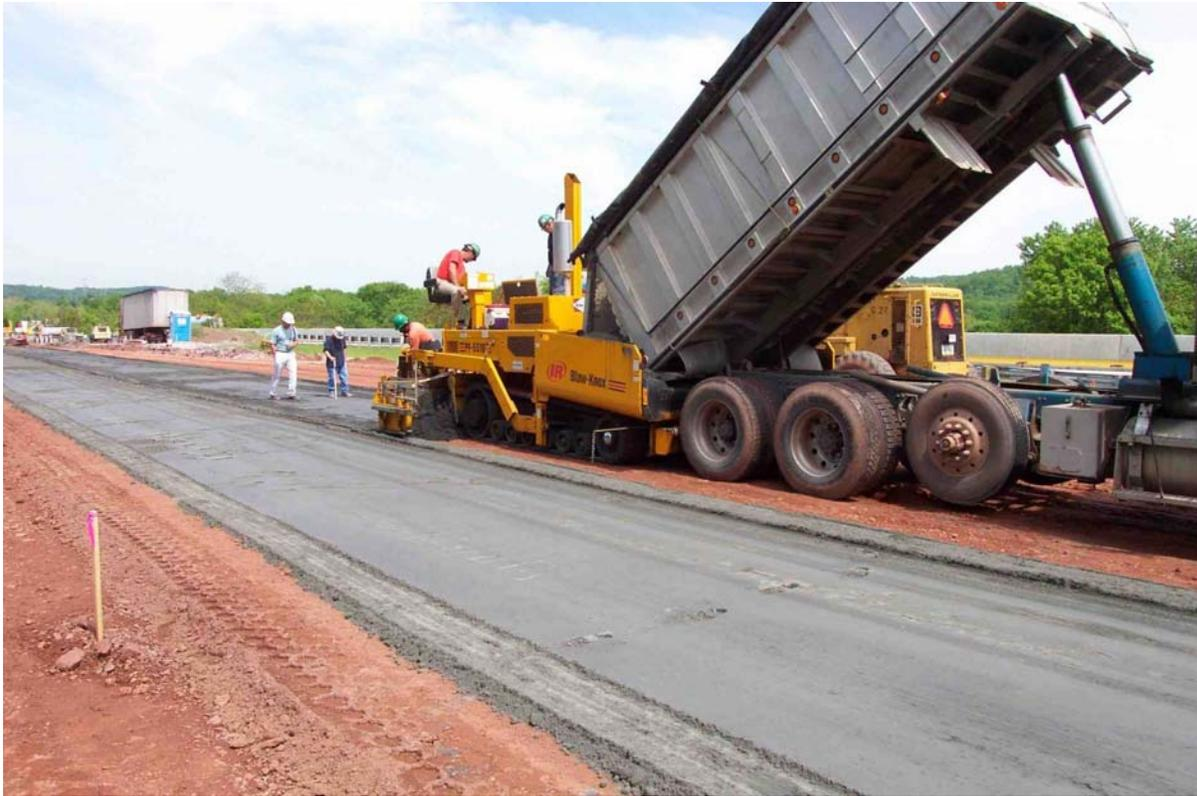
**Figure 2: Moisture-conditioned fly ash from the PP&L Brunner's Island Power Plant being applied at 6% by dry weight soil on PennDOT SR-283.**
