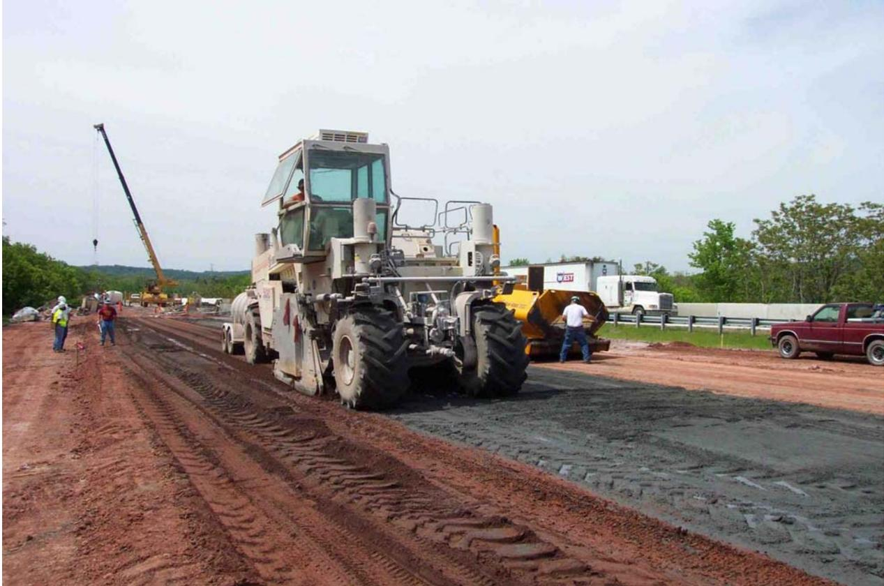
**Figure 3: On PennDOT SR-283, a “road reclaimer” mixes moist-conditioned fly ash from Brunner Island, PP&L plant near Harrisburg, PA, to a depth of 12 inches. Lime had been similarly added on the previous day.**
