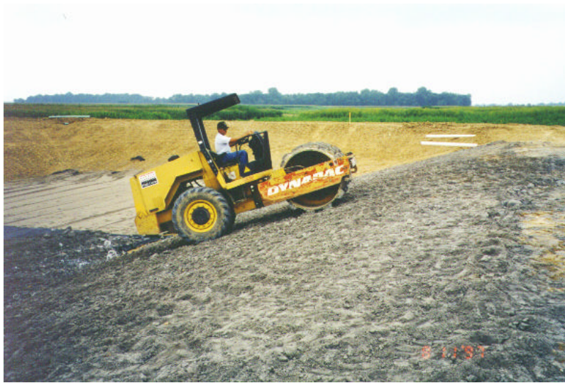
Figure 3. Compacting FGD Material on a Side Slope
