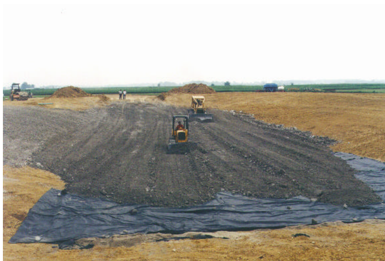
Figure 2. Spreading the FGD Material
