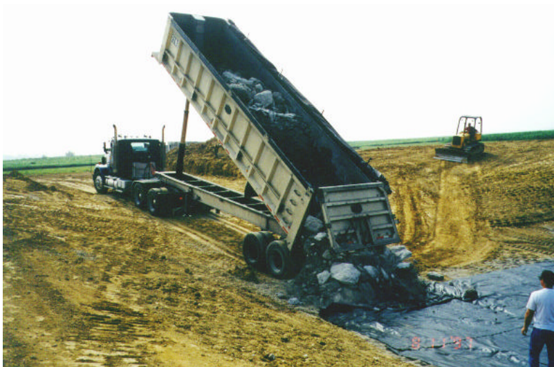
Figure 1. Truck Unloading FGD Material
