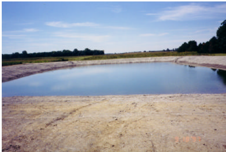
Figure 4 Facility Filled With Water
